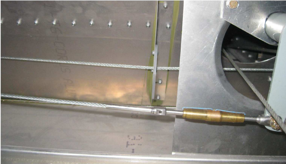
Above: Cable turn-buckle (for left-side aileron) in foreground ; aileron balance cable and fairlead above (in background)
