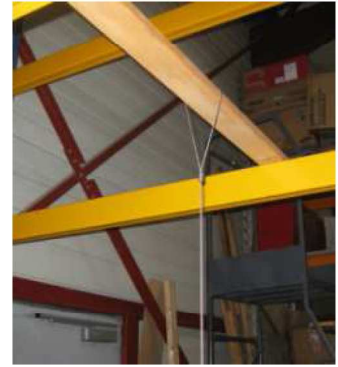
Detail: suspended cable with test weight.
