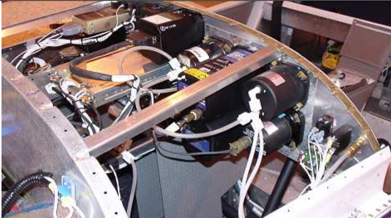
Typical installation of instrumentation
